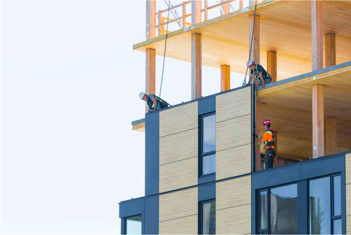
Figure 6. Construction of the Brock Commons student residence in Vancouver (UBC), the tallest cross-laminated timber (CLT) building in the world at 53m high. In many countries building regulations still limit the heights of timber buildings based on outdated regulations. Photo source: https://www.naturallywood.com/
