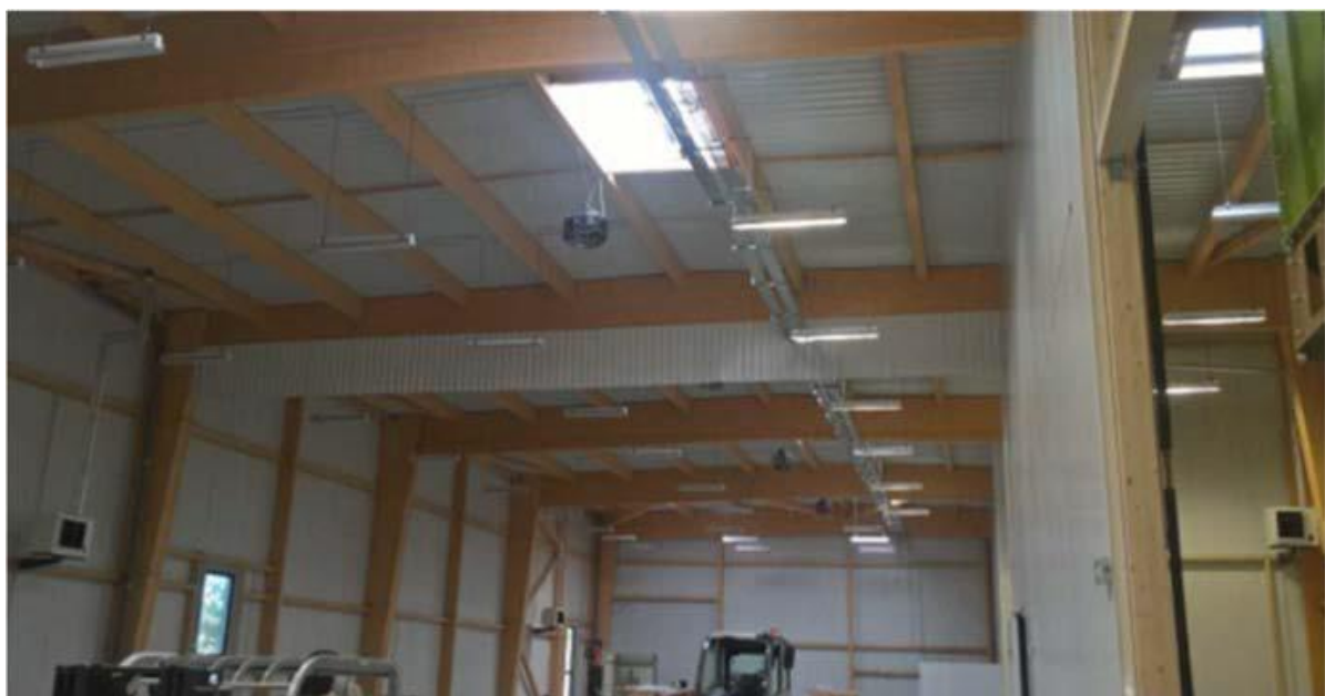
Figure 3.1. The Industrial building with glulam beams, located in Pessac, Nouvelle Aquitaine.
