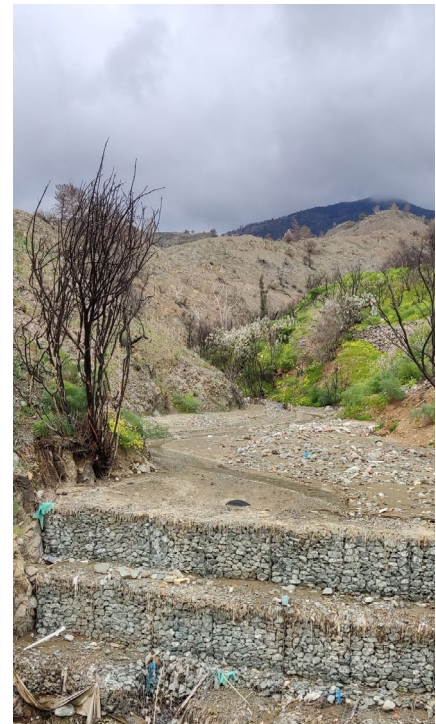
Accumulation of materials in the gabion dam from the upper part of the basin. Kostas Aristeidou, © courtesy of the Ministry of Agriculture, Rural Development and Environment of Cyprus.
