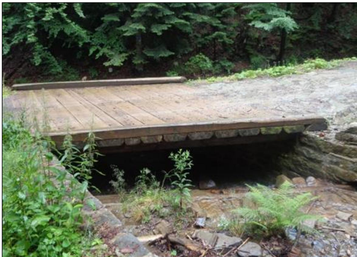
**Figure 31.** Wooden bridge more user friendly to aquatic organisms replacing concrete culvert.
