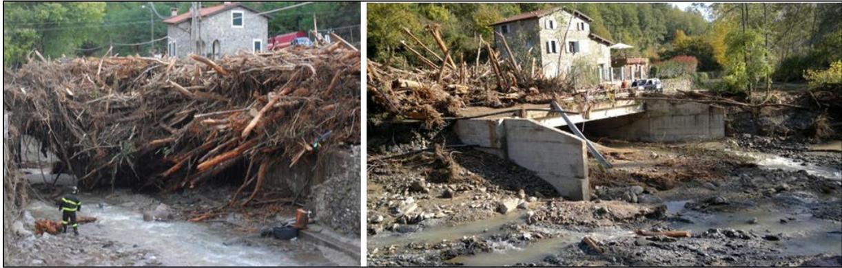
**Figure 13.** Examples of bridges clogged by LW transport during the October 2011 flood in the Magra River catchment (photos courtesy of the Province of La Spezia).
