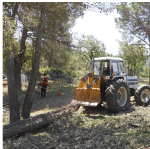
Perimetral security strip under execution. Source: DIBA
