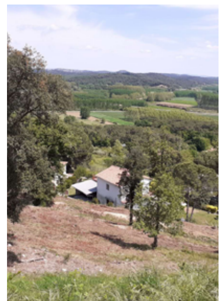
Example of a residential area in Barcelona province where a perimetral security strip is applied. Source: DIBA
